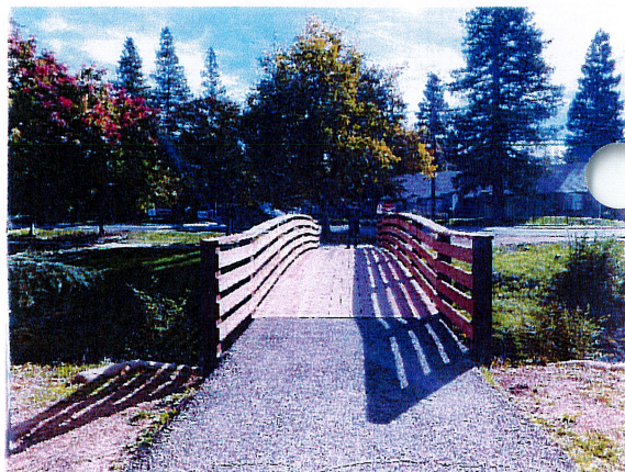
New bridge at Howe Park
